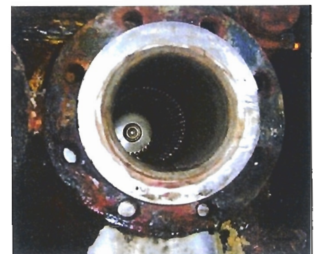
Scale-free after the Hydroflow treatment
