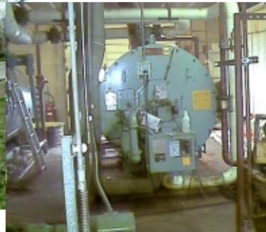
Akron Baptist Temple, Akron, Ohio Heating boilers: York Shipton 2 stage Controls: Honeywell/Johnson
