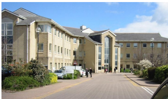
Typical building using steam generated humidifiers Orange Telecomms. SJames building Bristol
