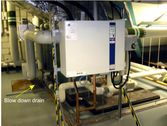
Typical stand-alone steam generator type humidifier unit. This model - ElectroVap MC has 2 steam vessels producing around 44kg of steam per hour.
