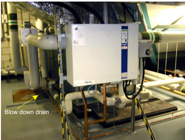
Typical stand-alone steam generator type humidifier unit.
