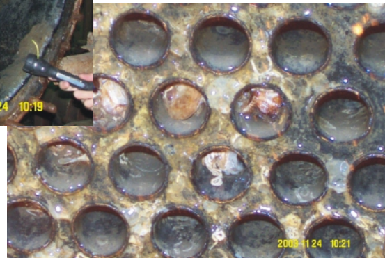
Exploded view of fouled heat exchanger before HydroPath
